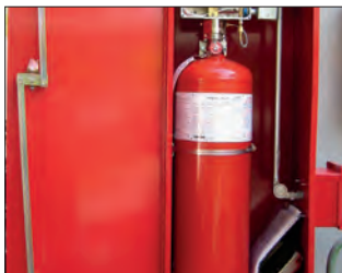
Integral dry chemical fire suppression
